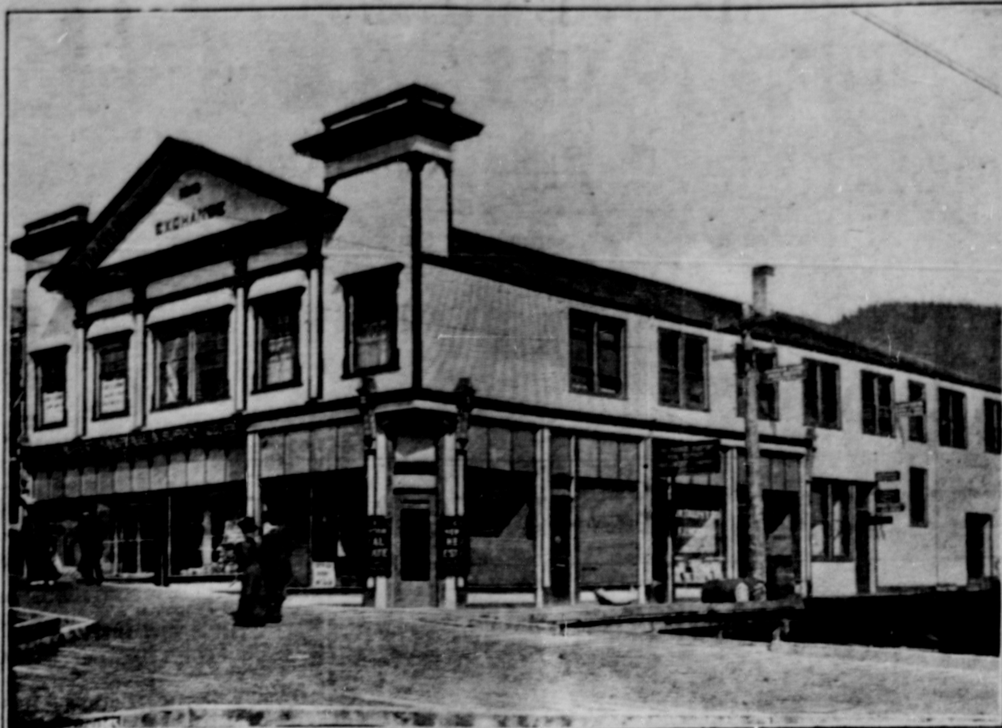
At Sixth Street and Third Avenue Crossing Where the Crowds do Congregate and Where the new Crossing Sweeper Brigade is Most Particularly Needed When It Rains
