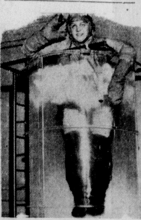
SWIZZLE STICK- Looking like a human swizzel stick in a giant-sized highball, Melvyn M. Maki, is shown as he demonstrated the navy's new submersion suit in a 32-degree tank of ice water in New York. The suit is fabricated of nylon coated with vapotex, and will allow Melvyn to spend three hours in the water. Ordinarily he'd freeze to death in 30 minutes.
